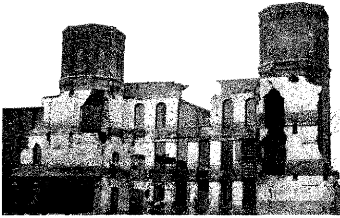
LAWRENCE MANUFACTURING CORP. Above left: View from behind the 1855 stair-tower unit. Note the absence of stairs, and the now-visible rectangular holes in which floor beams rested as part of the "slow-burn" construction. Above right: View from the roof of the remainder of the river mill reveals still-smoldering charred timbers amidst the ruins of one stair-tower and adjoining wall (left), the water-closet tower (center), and the 1835 cotton storehouse beyond. A crane works to demolish unstable walls. Laurence Gross photographs for Museum of American Textile History.
