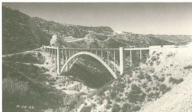
PINTO CREEK BRIDGE (1949, Ariz. Hwy. Dept., 371-ft. span) in Gila Co., photographed at completion. It is one of 15 steel arches in the inventory, which was extended into the 1950s to include all examples of this type. ADOT photograph.
