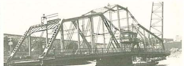
THE CUYAHOGA AND ITS BRIDGES. Above: Panorama from high in Terminal Tower reveals the river's tortured course through the Flats. Left: A majestic pair of early 20th-C, rolling-lift bascules. Right: Center Street Bridge (1901, King Bridge Co.), Cleveland's last remaining swing bridge. R. Frame photographs.
