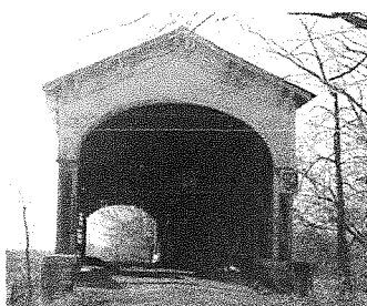
SMITH BRIDGE (1877), a single-span, Burr truss over the Flatrock River in Rush Co., Inc. Russell Dougherty photograph.
