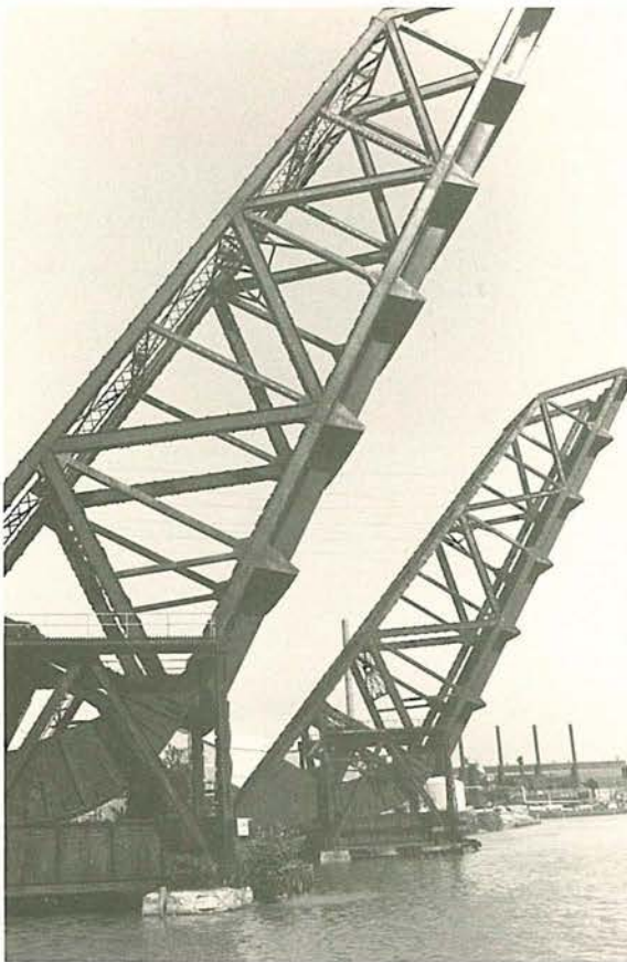
THE CUYAHOGA AND ITS BRIDGES. Above: Panorama from high in Terminal Tower reveals the river's tortured course through the Flats. Left: A majestic pair of early 20th-C, rolling-lift bascules. Right: Center Street Bridge (1901, King Bridge Co.), Cleveland's last remaining swing bridge. R. Frame photographs.
