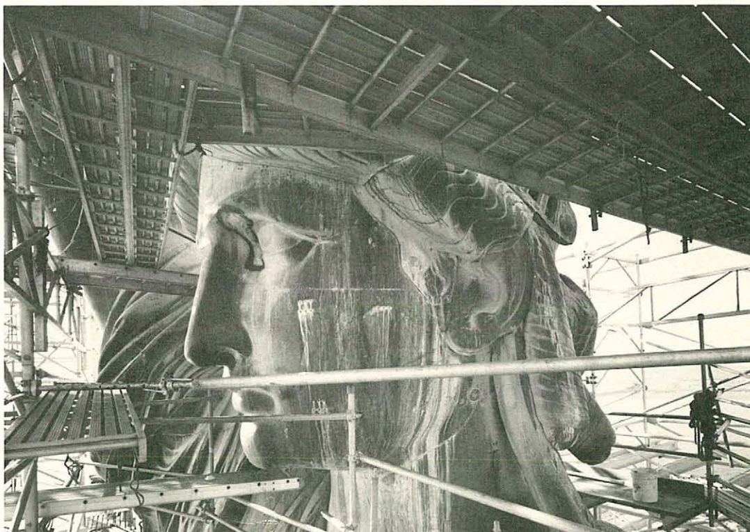
Liberty's magnificent head. The dark area at the eye marks a graft of new copper skin. The lobe of the nose also has been repaired. Streaks on the face and neck were caused by a bicarbonate-of-soda solution, used to remove coatings on the interior surface, which oozed through joints between copper plates and through the holes for rivets connecting the skin with iron support straps on the inside. Jet Lowe photograph for HAER (12-85).
