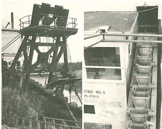
GOLD DREDGE 8, Fairbanks, Alaska. Each manganese-steel bucket weighs 1,583 lbs. and has a 6-cu.-ft. capacity. ASME and Fairbanks Convention & Visitors Bureau photograph.
