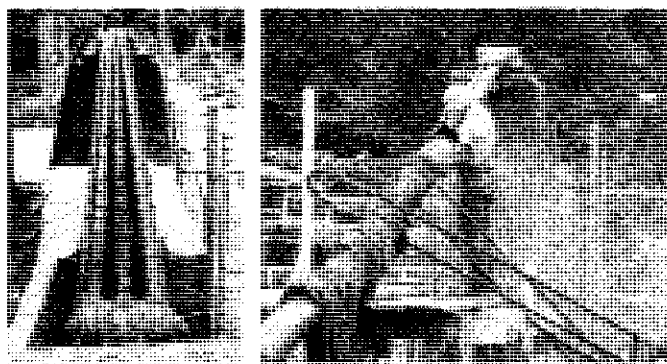
THE DELAWARE AQUEDUCT. Above far left & right: The upstream and downstream faces, looking toward N.Y. Above left center: Repairing the upstream pier faces by repointing the joints and replacing missing stones with originals found in the river. Above right center: Installing a wooden icebreaker. Below left: Cable at an anchorage. Below right: Sandblasting off the rust, old paint and oil. Center-left photograph by Robert M. Vogel; other photographs by Sandra Hauptman.
