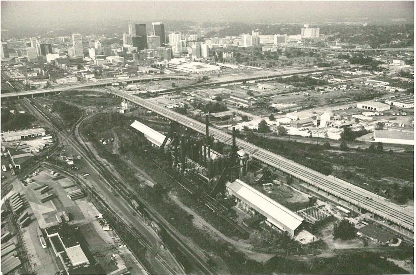
SLOSS FURNACES NATIONAL HISTORIC LANDMARK. The Sloss complex is located about a mile from downtown Birmingham (visible in the distance, at the top of the photo). Sloss has two blast furnaces, which were supported by the dark cluster of auxiliary equipment at the site's center. A long, white-roofed cast shed extends out from each furnace. Only the east half of the complex (the furnace and cast shed nearest the photo's lower edge) is interpreted and open to the public. Sloss Furnaces photograph.
