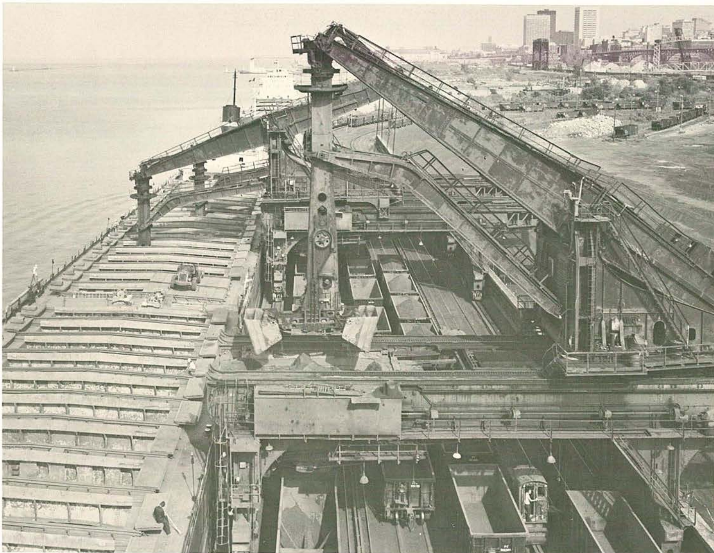
Hulett ore unloaders (above & below), Pennsylvania Rwy. Ore Dock, Cleveland. Jet Lowe photographs for HAER.
