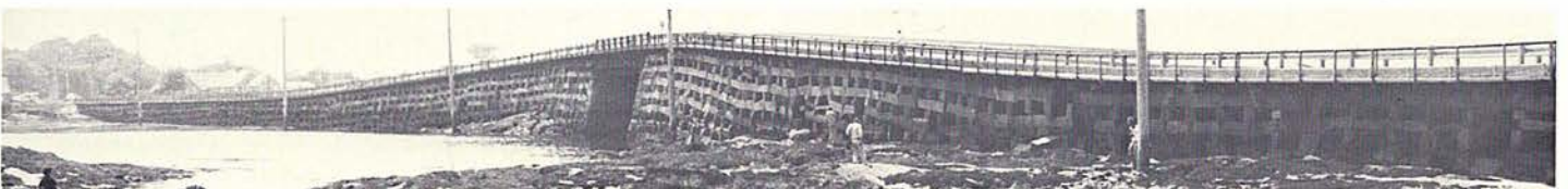
Below: Bailey Island Causeway (1928), a granite-slab crib bridge between Bailey & Orrs islands, Casco Bay, Me. Left: Neil Cossons, Maritime Museum director, Greenwich, stands amongst the Bailey's cribstones. R.M. Vogel photographs.
