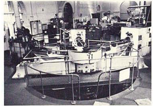
EAST BOSTON SEWAGE PUMP-ING STATION: E.P. Allis horizontal triple-expansion steam pumping Engine No. 3 (1899), one of two extant here. Operated during special pre-conf. tour on Thursday. Richard Hills photograph.
