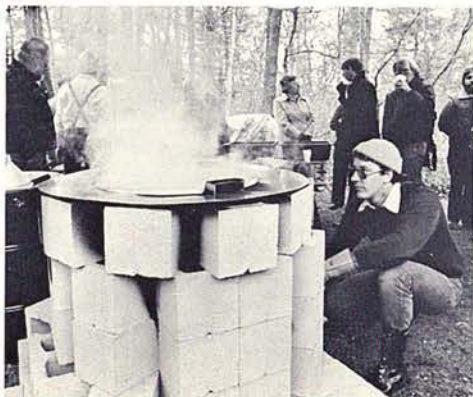
Gare Reid, Kendall Whaling Museum manager, fuels the fire of the analog try-works which is designed to produce whale oil from blubber. B. Bailey photograph for Kendall Whaling Museum.
