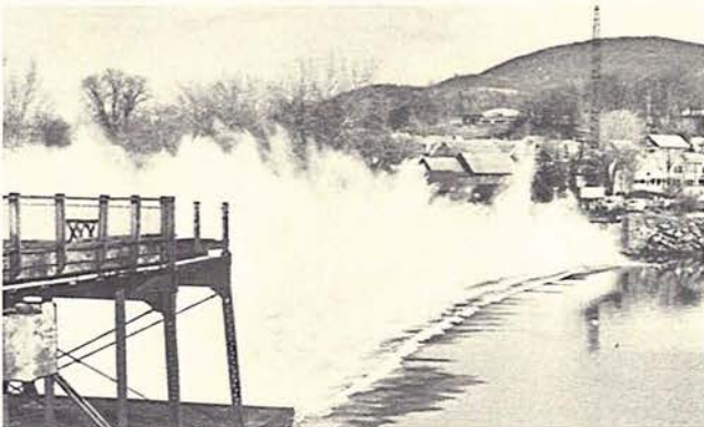
Stubborn bridge: The Bellows Falls Arch Bridge, spanning the Connecticut River between Walpole, N.H., and Bellows Falls, Vt., withstood four blasts from explosives before finally being downed with the aid of welders' torches last Dec. Wide World Photos.
