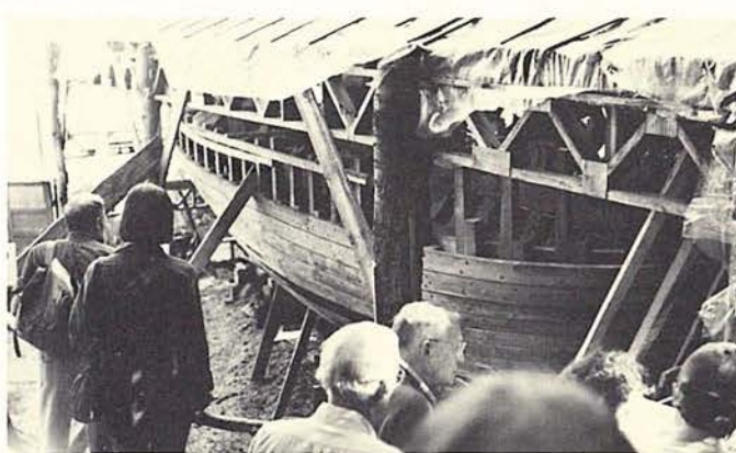
Outside the Apprenticeshop, tour members examine construction of a "pinky" of late-18th c. design.
