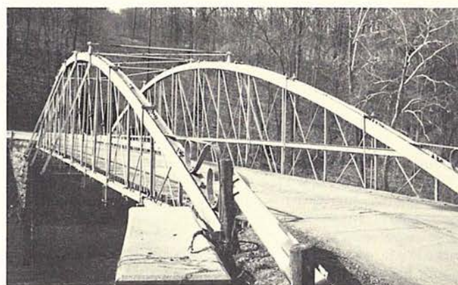
King patent bowstring arch bridge (1871), spanning Todd's Ford Creek in Warren Co., Ohio, prior to being dismantled last year. David Miars photograph.
