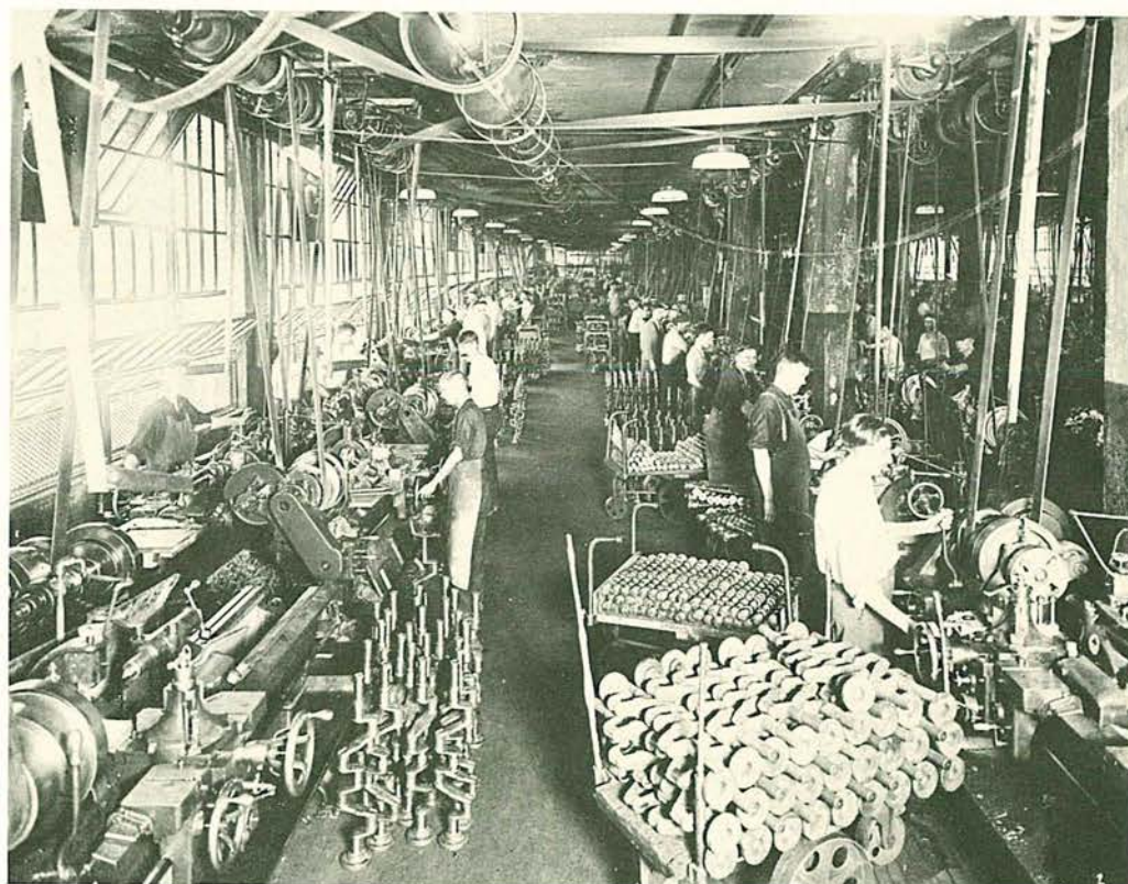
Machine shop, crankshaft and camshaft manufacture, Dodge Main, 1915. Chrysler Corp. photograph.
