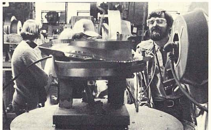
The ever-curious Mike Folsom observes the button-blank hopper feed at the Ball & Socket Mfg. Co., Cheshire.
