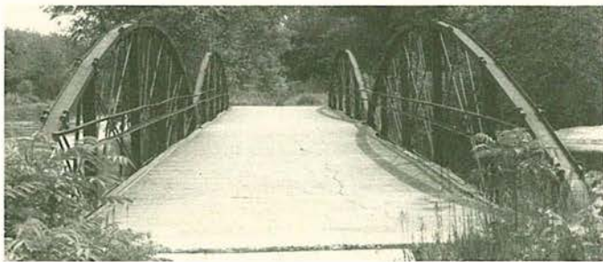
Double-span bowstring arch truss, La Crosse Co., Wisc. Historic Preservation Divn., State Historical Soc. of Wisc. photographs.
