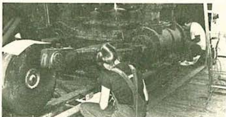
1979 IA Institute participants measuring a water-turbine-powered pumping engine of 1874. Vergennes, Vt. Jennifer A. Wilson photograph.
