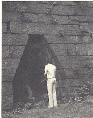
Measuring the tuyere at Horse Creek Furnace, Venango County, Pennsylvania. J. White photograph.
