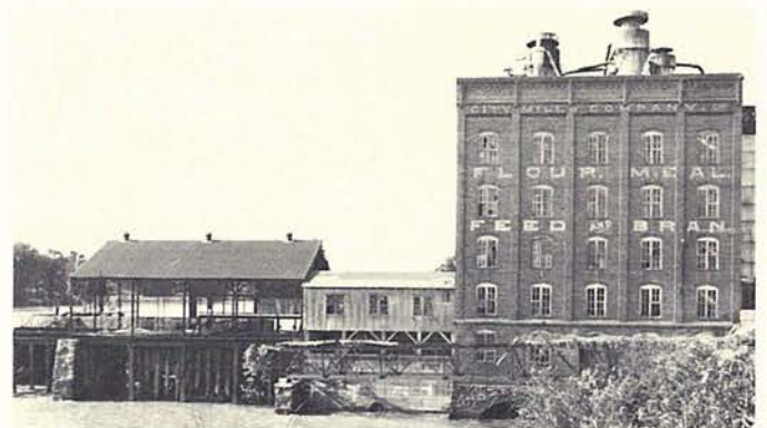
City Mills, downstream side. At the left are the remains of the Columbus RR Co. hydroelectric station (1894-96), largely dismantled in 1950; in the center the mill's wheelhouse containing three 62-inch Leffel vertical turbines; and at the right the flour mill of 1891.
