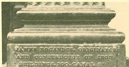
THE FIRST CAST IRON HOUSE ERECTED. ERECTED BY JAMES BOGARDUS, Builder of CAST IRON BUILDINGS and MANUFACTURER OF IRON AND STEEL. James Bogardus' cast-iron "house" erected 1848 at Center & Duane Sts., N.Y.C., generally acknowledged by historians to be the first in the world and absolutely claimed by Bogardus to hold that priority: if not inscribed in stone at least cast in iron (pilaster base, commercial building, Cooperstown, N.Y.) Lithograph, Museum of the City of N.Y.
