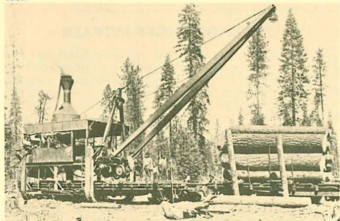
A McGiffert Log Loader at full cry—toes down, wheels up empties at ready. From Clyde Iron Works catalog , Natl. Museum of History & Technology.
