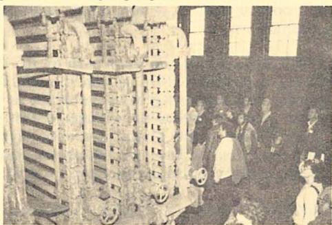
Merchants' Cold Storage Warehouse—refrigeration condensor coils, the point at which the heat taken from the cooled substances is removed from the system.
