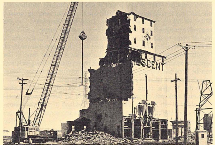
Crescent "H" Elevator, 1899, in the traditional heavy-timber-frame-and-corrugated-sheathing mode.
