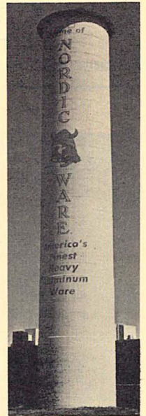
Peavey-Haglin experimental Concrete Grain Elevator, 1899-1900. Ht.: 125 ft. Interior diam.: 20 ft. Walls: 12 ins. at base, tapering to 8 in. at top.
