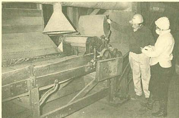
(L) Alfalfa cutter at Byfield Snuff Mill. (C) Bruce Tompkins, Prop. of Daniels Wagon Works, operating a chisel-type hub mortiser. (R) the works-built felloe bender at Daniels. At center is the former against which the felloes are bent. Jonathan Woodman photos.
