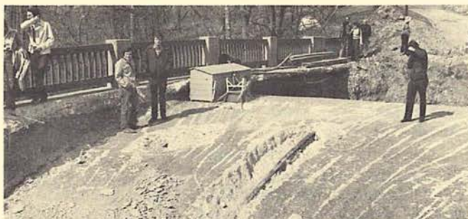
AS THOUGH FOR THE OCCASION, the spandrel filling of the Eden Park Bridge had been removed and one of the 9-inch reinforcing I-beams exposed. This was the third American bridge built on the Melan system (1895), in which curved, standard beams were used to reinforce a concrete arch of relative thinness.
