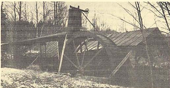
ADIRONDACK SAWMILLS. Above: One of the surviving machines in Emerson's Sawmill. The diamond windows result from the extensive diagonal knee-bracing in the frame. Below: the steel wheel of Kilmer's Mill. Peter H. Stott photographs.
