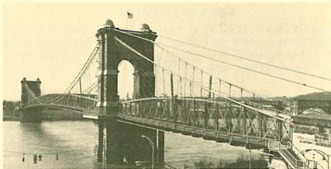
WHILE THE ELEGANCE of Roebling's Covington & Cincinnati Bridge was severely diminished by the deep steel trusses and additional main cables added in 1898, it survives in full service as a masterwork.
