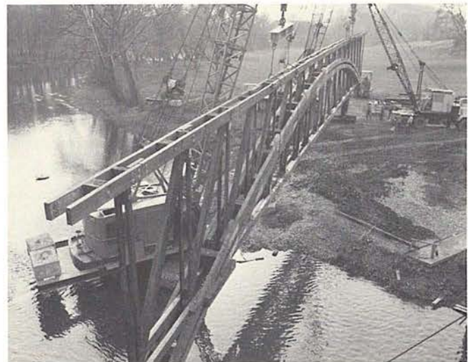
Hunsecker Bridge. Framing complete and sheathing begun (above); one truss being hoisted into place (below). Penna. DOT photos.
