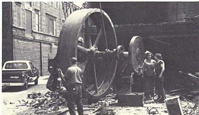
The Slater Mill Harris-Corliss engine flywheel, crank, &c, leaving.
