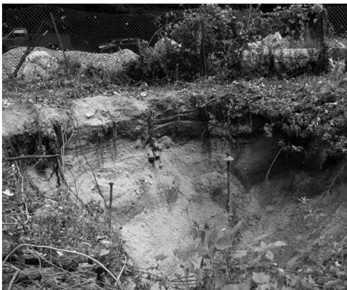
The 15-ft.-deep cave-in exposed metal rods that may have braced the timbers of a trestle that predated the tunnel.
