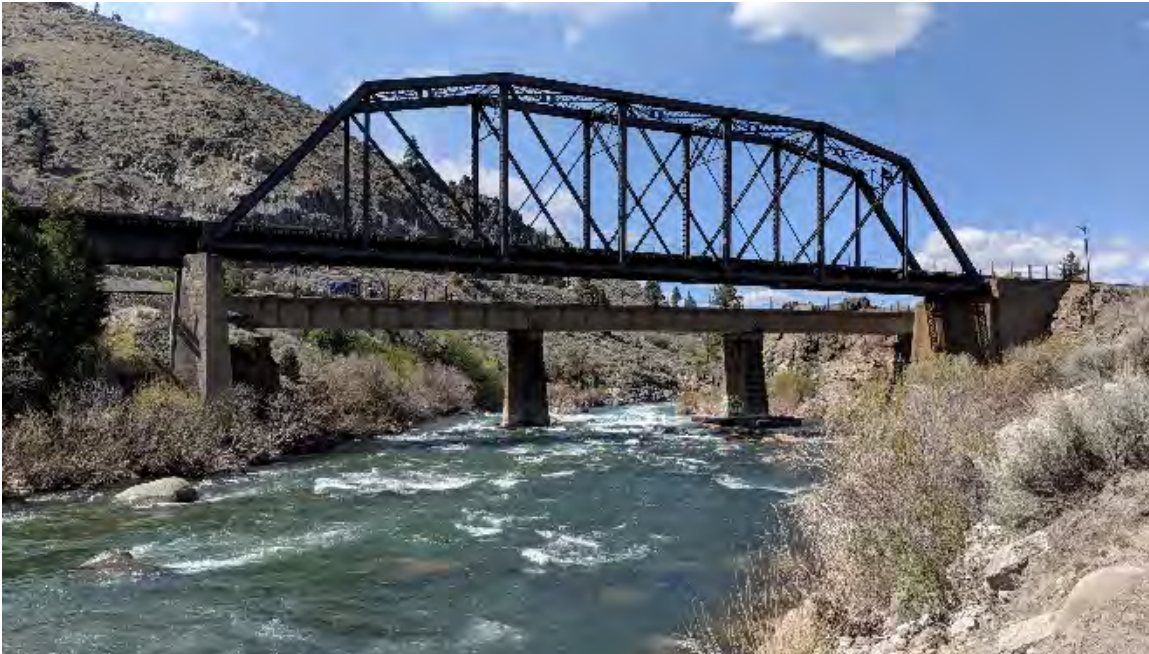
1907 truss and 1915 girder SPRR bridges crossing the Truckee River at Fleish (MB)
