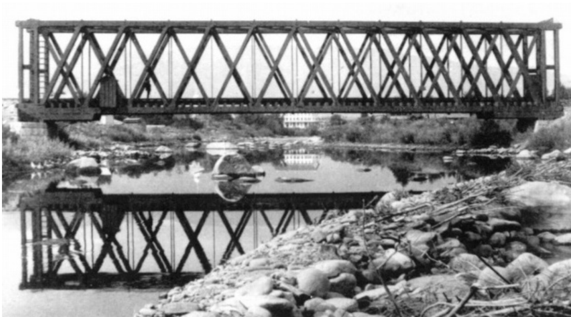
V&T RR Bridge over Truckee River, Reno, 1880. The timber Howe truss was replaced in 1896. (WNHPC)
