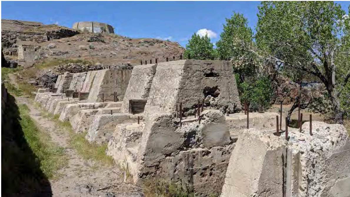
Remnants of the Nevada Mining Reduction & Power Co. Concrete stamp battery foundations and cistern in the distance. MB)
