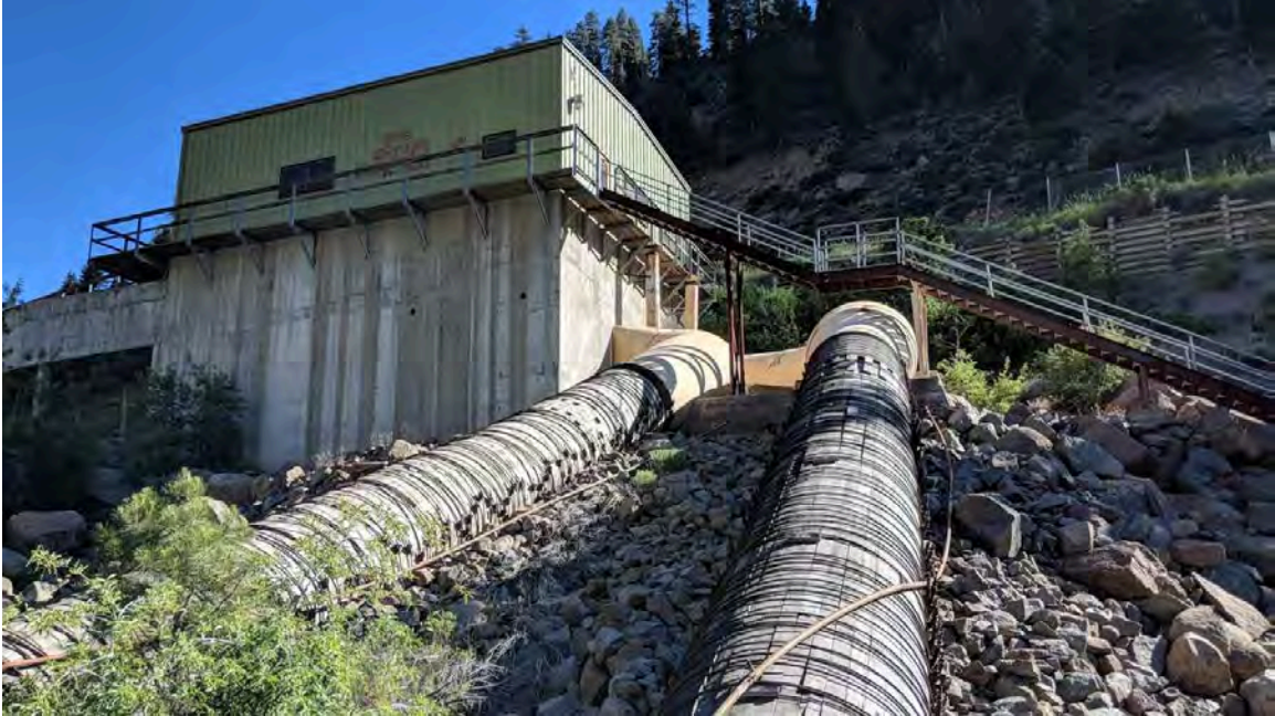
Farad intake building and wooden penstocks (MB)
