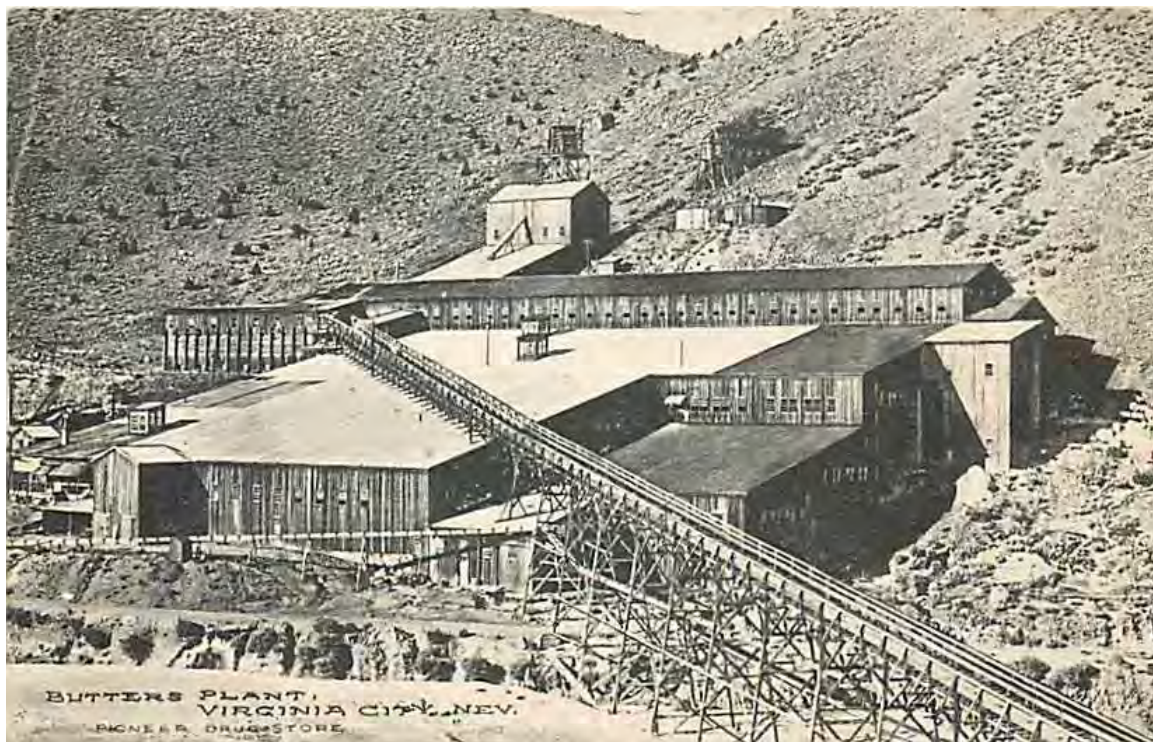
View of the Butters Plant with the wooden flume from the Kinkead Mill (ALB)
