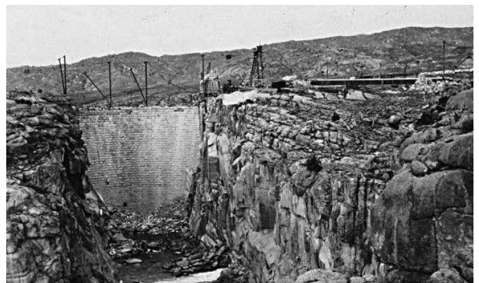
Construction of the Pathfinder Dam, c. 1908.
