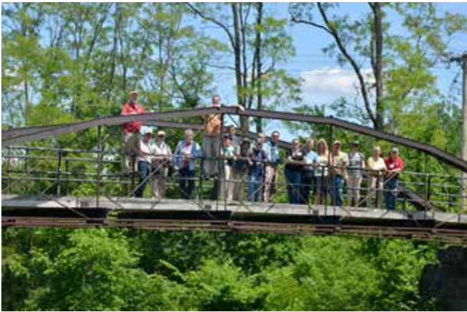
Vischers Ferry Bridge, a Whipple bowstring of 1869, gets some love from the SIA bridge tour group.
