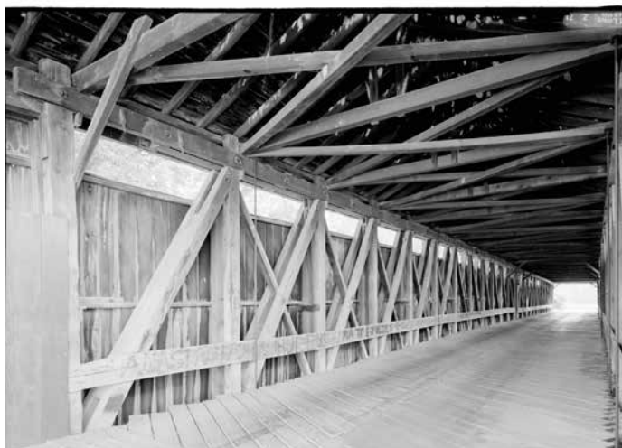
Eldean Bridge, vertical and diagonal endpoints at east portal, 2002. HAER OH-122-10.
