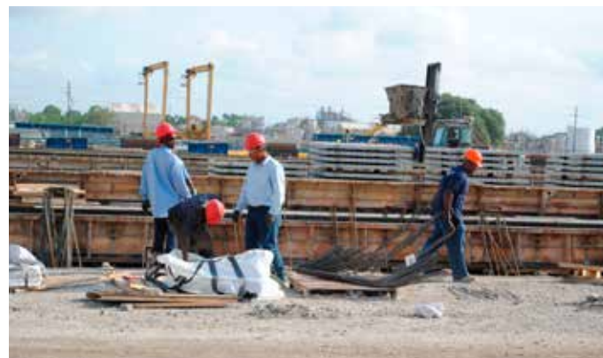
The casting line at Flexicore of Texas.
