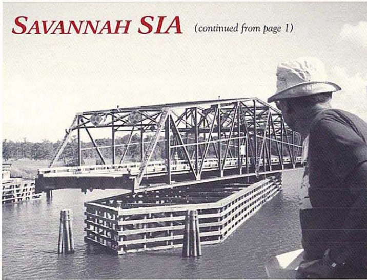
The Houlihan Bridge (1954), a swing span, was opened by special arrangement with Georgia DOT for the SIA's riverboat tour.
