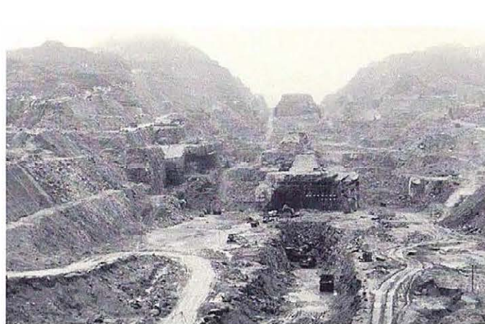
Excavation for the ship locks dwarfs the earth-moving equipment at the Three Gorges Dam near Yichang.
