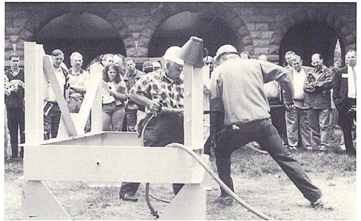
Pneumatic riveting was demonstrated at the bridge workshop.
