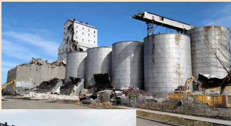
Electric Steel Elevator, Apr. 7, 2017. Remaining are a row of Turner's original 80-ft. steel tanks (1901, 125,000 bushels), a row of 65-ft. steel tanks, (1903–1906, 100,000 bushels), and the all-steel headhouse.
