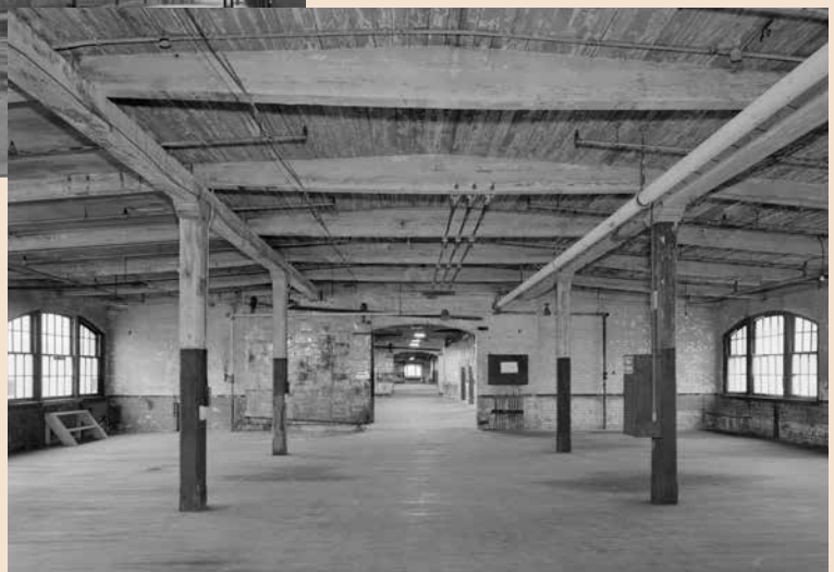
Ford Piquette Plant, second floor interior, Ford engine cutaway and mill construction, ca. 1968.
