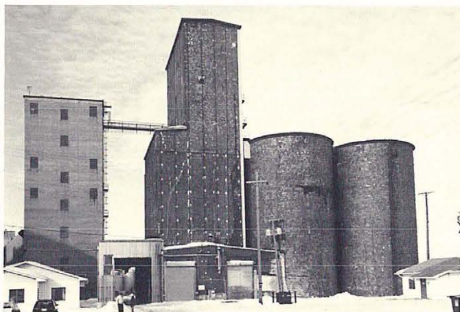
the 1887 Globe Elevator, perhaps the nation's oldest standing wood-cribbed terminal elevator; and the Great Northern Elevator (1901), a rectangular-bin steel structure engineered by Max Toltz and a sibling of Buffalo's landmark Great Northern Elevator (1897-98; also viewed in 1992). R.M.F.
