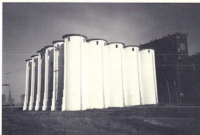
Above: On the Duluth side stands the nation's first full-scale, operational, cylindrical reinforced-concrete elevator, built by the Peavey Co. in 1900.
