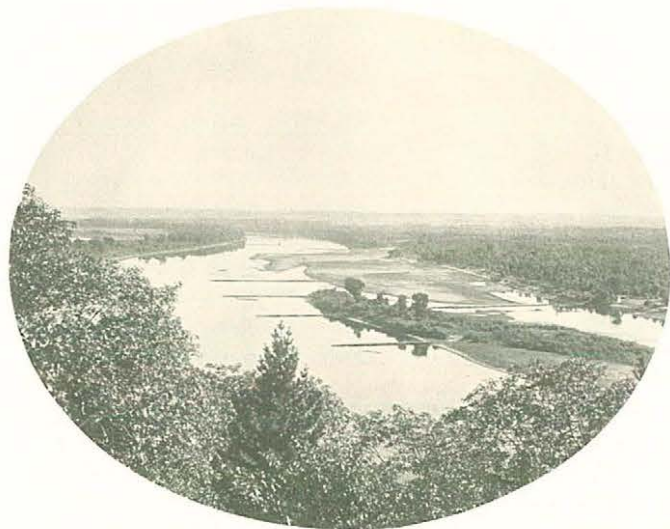
The construction of wing and closing dams to improve navigation with a 4 1/2-ft. channel was a major Corps project on the Mississippi. In 1891 Bosse recorded the process ( above, left & right ) of building dams using baled willow brush layered with rock. Below left : The finished closing dam, anchored with pilings, at Otter Chute in 1889. Below right : The scene of Pine Bend in 1891 shows a completed set of wing dams forcing the water into a narrower, faster, and deeper channel.
