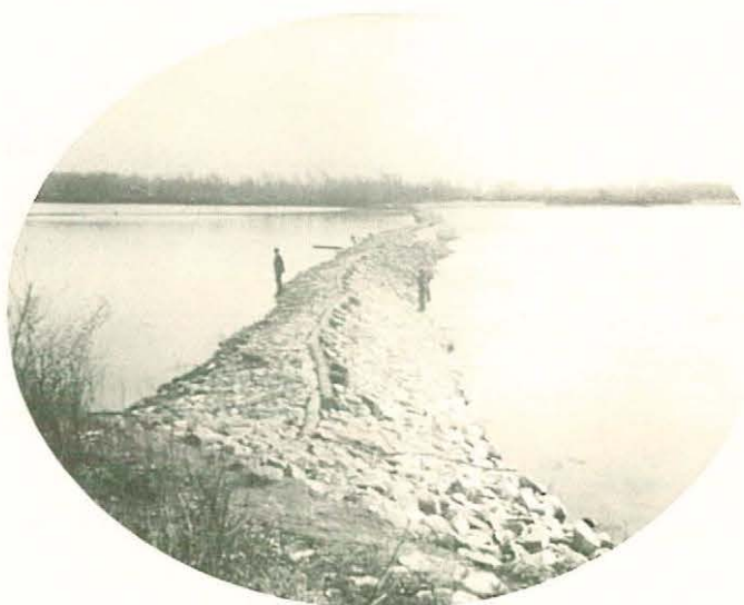
The construction of wing and closing dams to improve navigation with a 4 1/2-ft. channel was a major Corps project on the Mississippi. In 1891 Bosse recorded the process ( above, left & right ) of building dams using baled willow brush layered with rock. Below left : The finished closing dam, anchored with pilings, at Otter Chute in 1889. Below right : The scene of Pine Bend in 1891 shows a completed set of wing dams forcing the water into a narrower, faster, and deeper channel.
