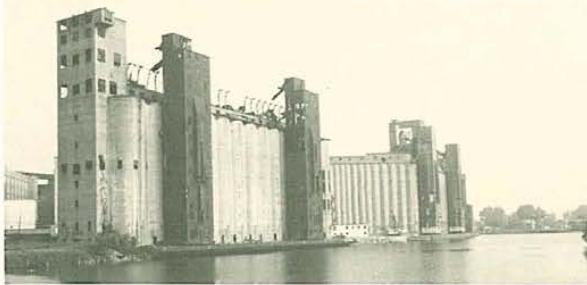
Grain elevators (clockwise from left): 1925 Marine A, inactive (L), & 1927 Lake & Rail, active (R); 1897 Gt. Northern with Pillsbury mill; GN's marine leg: circular reinforced-concrete marine tower (1911, 1st on Gt. Lakes) at Frontier Elevator; "tripper" (unloads grain from conveyor into bins) in Koch Malting elevator. R. Frame photos.
