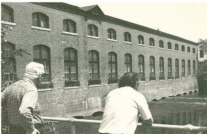
Mechanicville Hydroelectric Plant (1897). R. Frame photograph.
