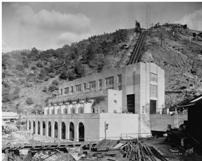
Big Creek Hydroelectric Plant, Powerhouse No. 3, construction photograph of 1923.
