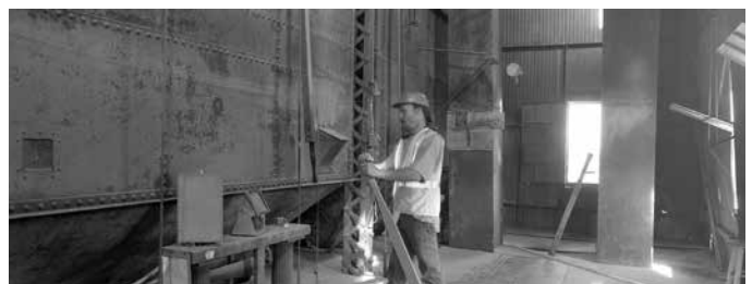
Electric Steel Elevator, interior.
