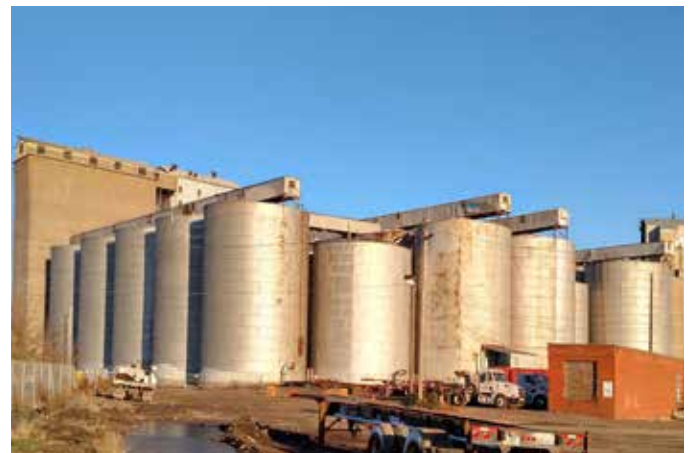
Electric Steel Elevator, Nov. 2016.
