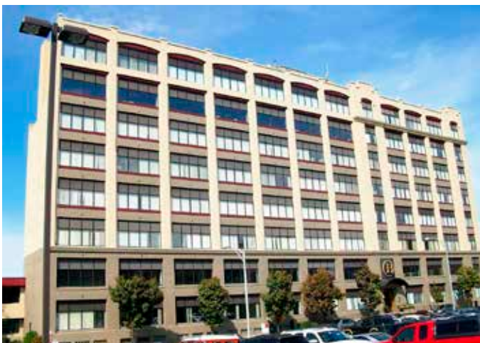
Cluett, Peabody & Co., now Hedley Park Place, 433 River St. (converted to offices).
