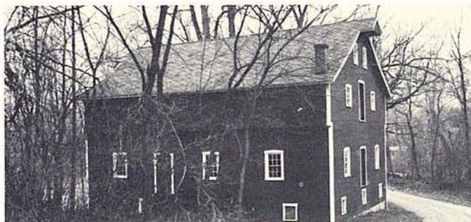
Gristmill (1818). Double overshot waterwheels have rotted away, although the shafts remain. Family tradition indicates that the top story was added after the initial construction. At right is the mill's "hopper boy". Invented by Oliver Evans, it was designed to cool and dry the meal after grinding. OHPO photographs.
