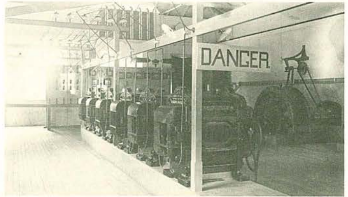
Interior view of the powerhouse with the air-cooled transformers in the foreground. In the background, one of the three generators (right) and the switchboard (left/center) may be seen. All electrical equipment for the plant was supplied through GE's Pacific Coast office.
