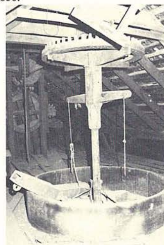
Saw frame and part of log-carriage feed mechanism. Donald Hutslar photograph. from a larger grouping that helped Ohio lead the nation in the production of corn whiskey in 1850.
