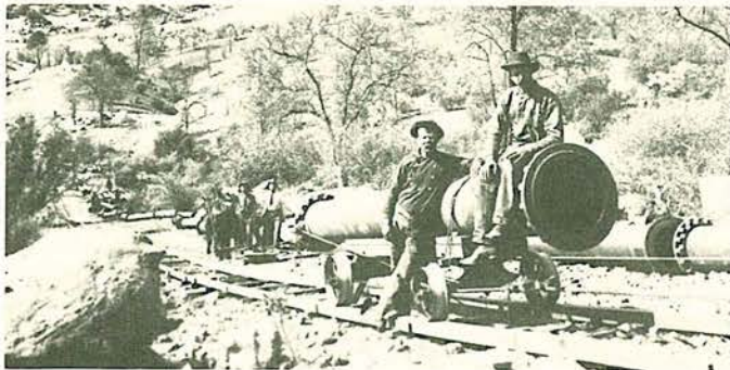
Work on the 4,200-ft. penstock stops for a short "photo break." Construction of the penstock had to be of high quality because of the great pressure exerted by a column of water 1400 ft. high. At the powerhouse, the water was under a pressure of 609 psi.
