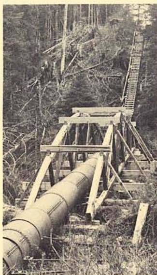
The Upper Salmon Creek plant receives water through this 30 to 40-inch, 4400-foot penstock. Small timber bowstring trusses carry the pipe across creeks. Stairs and handrail are provided on the steeper sections for the penstock is the path to the dam.
