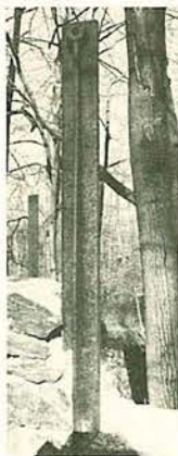
One of six cast-iron braces imbedded in the foundation wall, Harris Chemical Co. site. John P. McCarthy photo-graph.
