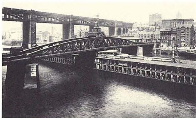
19th-century view of the Tyne Swing Bridge. The steam pumping plant is in the fender structure at the right. Behind is R. Stephenson's famed high-level railway & highway bridge of 1849. Both bridges are in full use today. Museum of Hist. & Tech. photograph.
