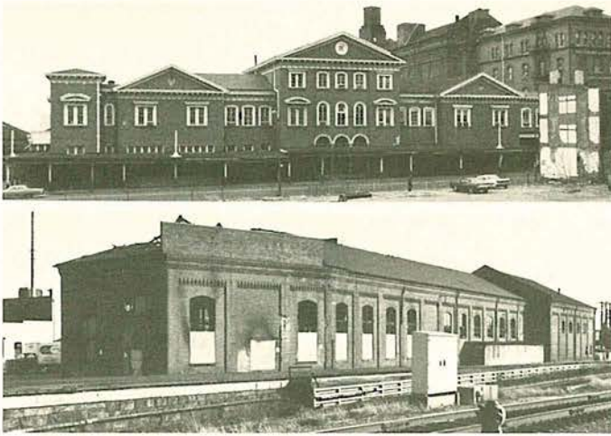
Top: Camden Station, c1855, earliest major urban RR station remaining in use in the U.S. Bottom: the B&O Belt RR Power House, built 1895 to furnish power for the first mainline RR electrification project. Engine room on left; boiler house on right.
