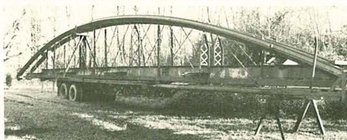
Wrought Iron Bridge Co. bowstring truss at Detour, Md., before and after the move to its new home.
