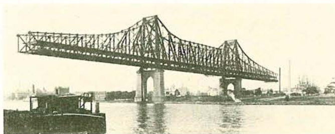
Top: Blackwells Island (Queensboro) Bridge, under construction, August, 1907. (If this doesn't explain "Cantilever," nothing can.) N.Y.C. Highway Dept. Colln. Bottom: Wurts Colln. view of H.C. Frick residence under construction, Sept. 1913. Both, Museum of the City of New York.
