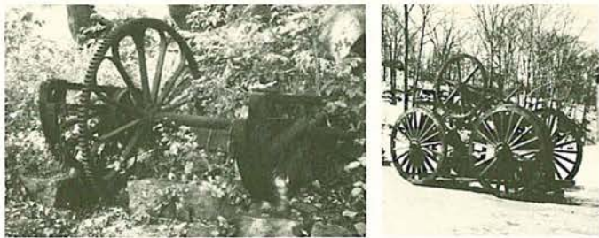
Quincy Granite Railway. (L) Ruins of one of the horse-drawn granite cars, with hoisting gear. (R) 1925 replica of same. Historic American Buildings Survey (c1936).
