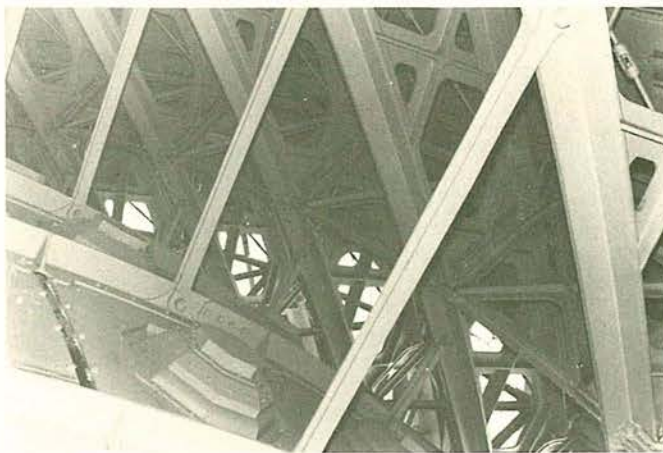
Between the Capitol domes. At lower-left the back sides of the octagonal coffers in the inner dome; above them the diagonal ties suspending the inner dome from the framing.
