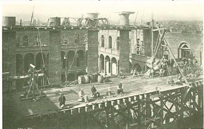
The Pension Building under construction, 1884. At center, one of the two ranks of mammoth brick columns rising in the court area. NMHT.
