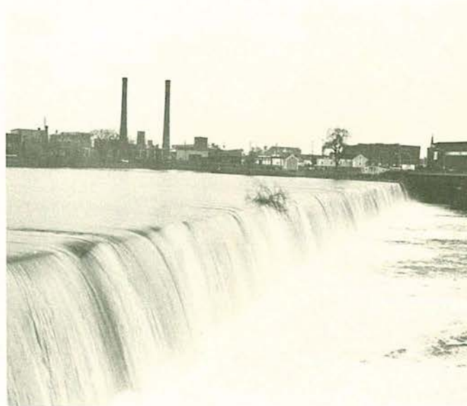
The Great Stone Dam across the Merrimack at Lawrence, 1845-48, providing a 30-ft head in the hydraulic canals on the N and S banks of the river. Peter H. Stott photograph.
