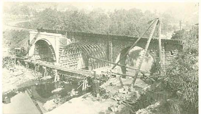
B&O's Potomac River crossing at Bloomington. 1916 photograph during widening to 4-tracks by application of Melan arches. B&ORR Collection, Natl Museum of History & Technology.
