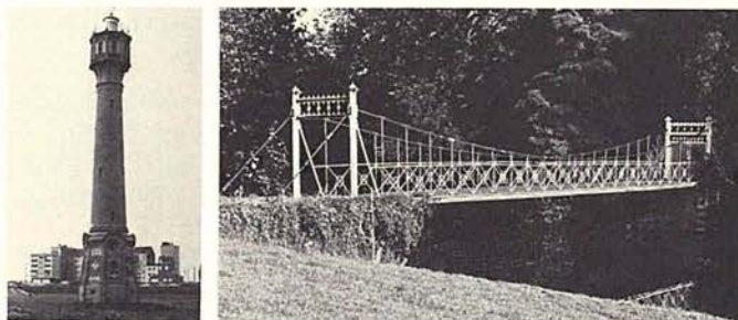
Belgian IA: Reinforced-concrete lighthouse at Heist, 1907, and the first Belgian suspension bridge, by Vifquin—c1825—possibly the earliest surviving on the Continent, at Bazel. A Linters
