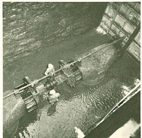
Dam 4 Hydrostation, 1909. L to R: The generators; one of the turbine drive sheaves & view up through ropeway; one pair of Leffel double turbines in dewatered wheelpit. Potomac Edison photos.
