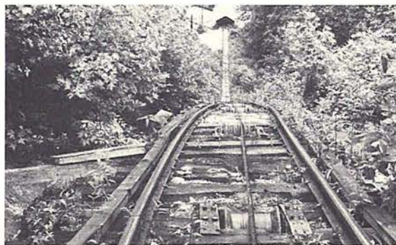
White Silica Sand Co incline, Lake City, Tenn., still in operation bringing sand from mountain-top pit to cleaning plant below. Operates on the balanced system with passing sidings at mid-flight. R L Johnson photograph.
