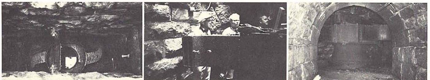
A feature of the Sept SIA Lehigh Valley Tour was a visit to the house of James Lee, formerly that of a Morris Canal plane tender, and access to the wheelpit housing the Scotch turbine that powered the plane [see "Oral History" above]. Left: the turbine from the ground surface, above. Center: the tangential spout of one arm. Right: the turbine seen from the tailrace tunnel (the vertical turbine shaft is missing). The water entered the turbine from below, through the pedestal.
