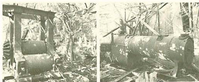
Three-roll sugar mill and Ames boiler, c1878, at Meyer Sugar Mill.
