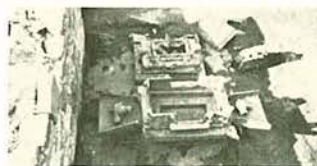
Forges found in the excavations of the Rogers Locomotive Co's boiler shop, 1873. A cleaned and reassembled forge in the foreground; one as-found behind. GFDC Photo by Lynda de Victoria [SIA].
