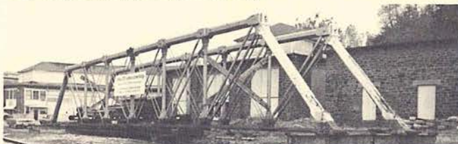
Lombard St. Bridge in transition. Top: the bifurcated "Water-pipe" center truss still in place spanning Jones Falls. Bottom: the two Pratt side trusses, having been lifted out intact, in temporary storage.
