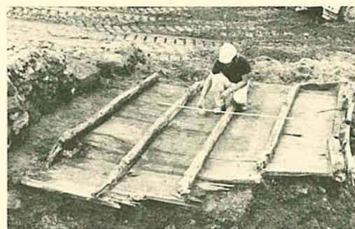
Right. Archeological observer Budd Wilson cleaning section of Morris Canal barge found during demolition of DL&WRR Station in path of highway construction. Remains of canal wall are at the left (6-ft. scale).
