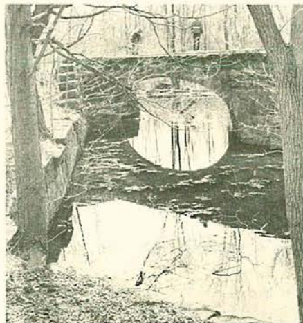
Masonry skew bridge spanning Canal at Lock 12 carried the parallel railroad that succeeded it. Photo: Thomas Pool.
