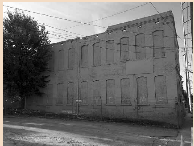
Trio dry cleaning building north façade with "Save Me" printed across the sealed windows.
