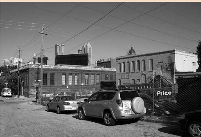
Trio Steam Laundry buildings. The c. 1905 plant (later Atlanta Brush Co., 19 Hilliard St.), shown left, and the c. 1910 expansion (20 Hilliard St.), shown right.
