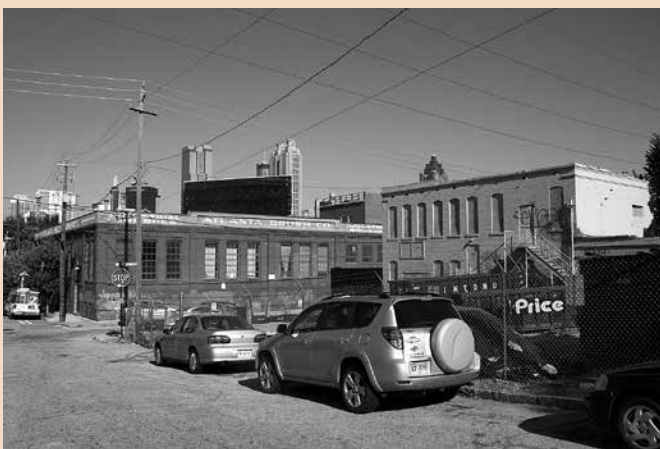
Trio Steam Laundry buildings. The c. 1905 plant (later Atlanta Brush Co., 19 Hilliard St.), shown left, and the c. 1910 expansion (20 Hilliard St.), shown right.
