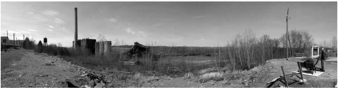
Huber Breaker, demolition nearly complete, Apr. 2014.
