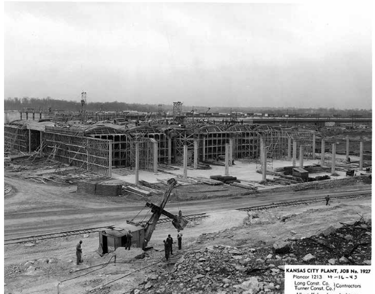
Pratt & Whitney Plant under construction in 1943.
