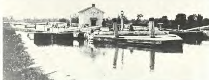
The lock-tender's house sits atop the Erie Canal's Lock 51 at Jordan, N.Y., in this c1895 view. The house looks much the same today. No. 51 is a limestone double-lock. Onondaga Hist. Assn. photograph.
