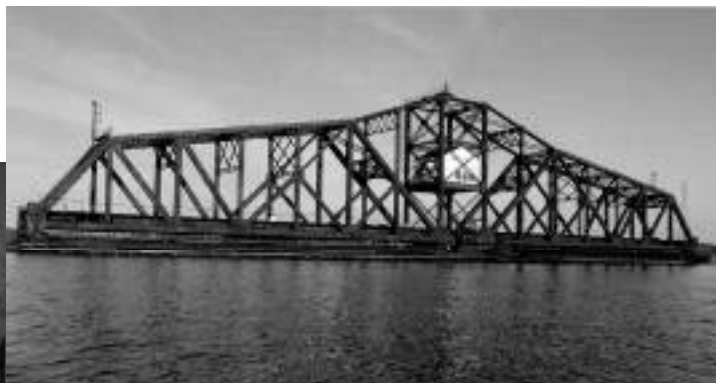
The Grassy Point Draw of the Burlington Northern RR built in 1887 by the St. Paul & Duluth Rwy.
