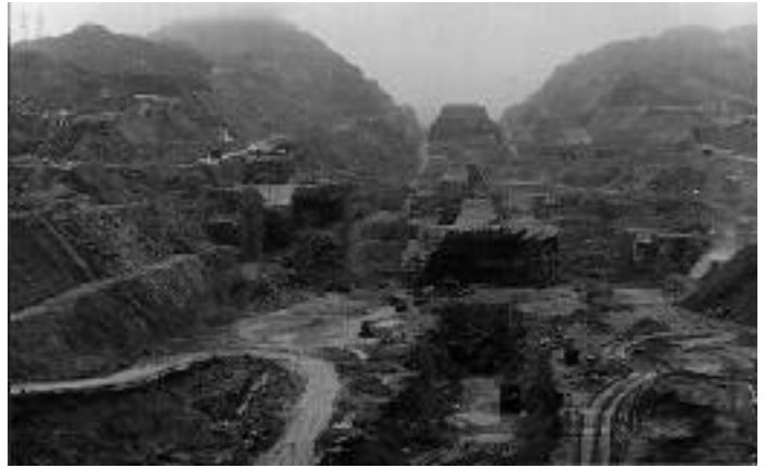
Excavation for the ship locks dwarfs the earth-moving equipment at the Three Gorges Dam near Yichang.
