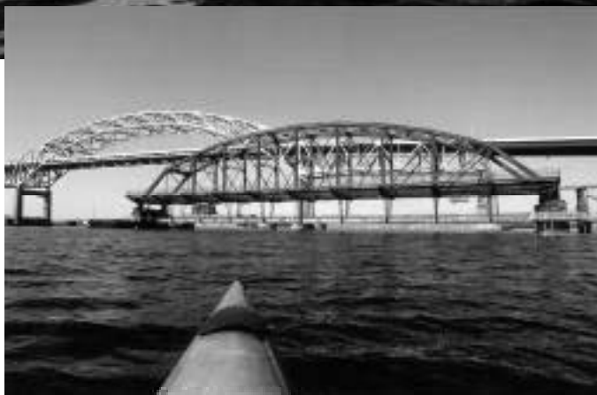
Interstate Bridge, originally known as the Duluth-Superior Bridge, was built by the Duluth-Superior Bridge Co., controlled by the Great Northern Railway, in 1897. Completion of the present High Bridge in 1961 (visible in background) eventually brought about the older bridge's closure. The draw span was pulled out in 1972 with only the Parker through-truss approach span remaining.
