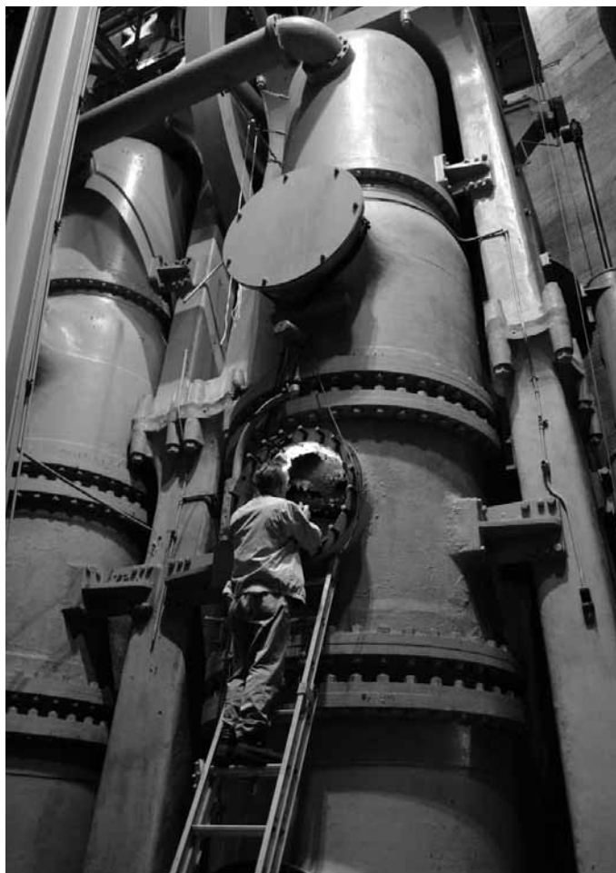
Upriver Tour participants had the opportunity to look inside the valve chamber of a pump at the Old River Station. The pumps are located about 100 ft. below ground level. Access was down by elevator, then up about 12 feet by ladder.
