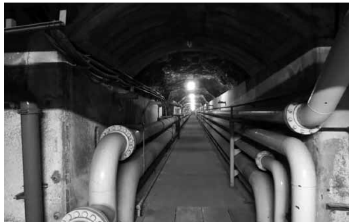
The cylindrical horizontal steel tanks at Has Saptan are connected to a series of underground tunnels housing the pipes connecting the tanks to Malta's ports.
